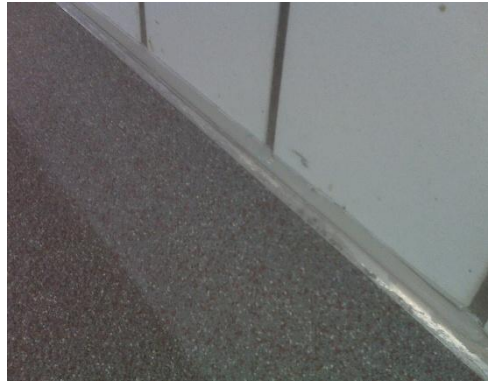
Finished cove molding with profile
